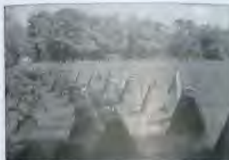
A short stop to inspect the "Dragon's Teeth" installed along the West Wall (Siegfried Line) Holland to Switzerland.
