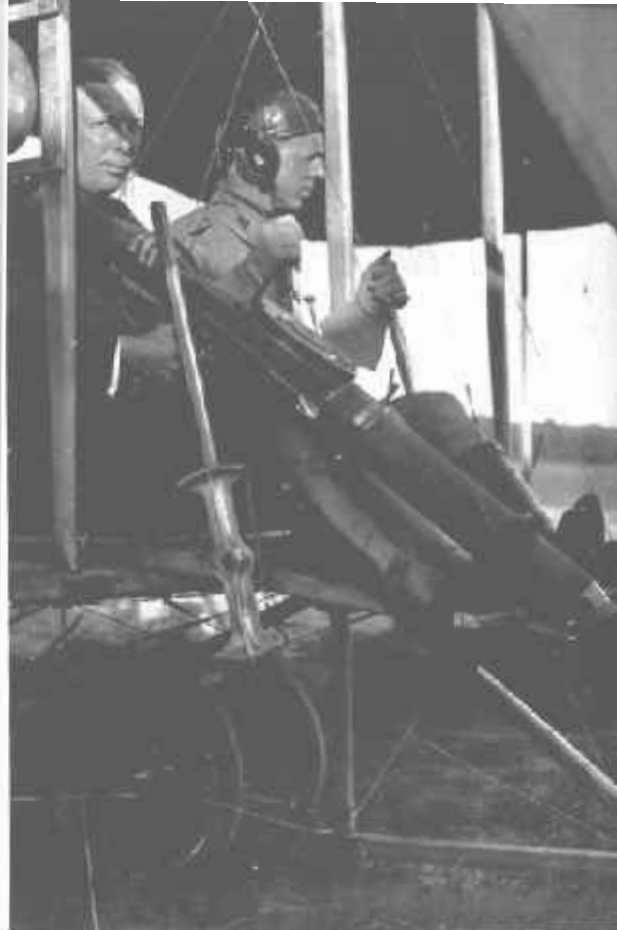
Captain C. Del. Chandler and Lieutenant Roy T. Kirtland—in Wright Type B airplanes with Lewis machine gun. June 7, 1912.—The first machine gun ever fired from airplane (Lieutenant Kirtland was pilot for test).
