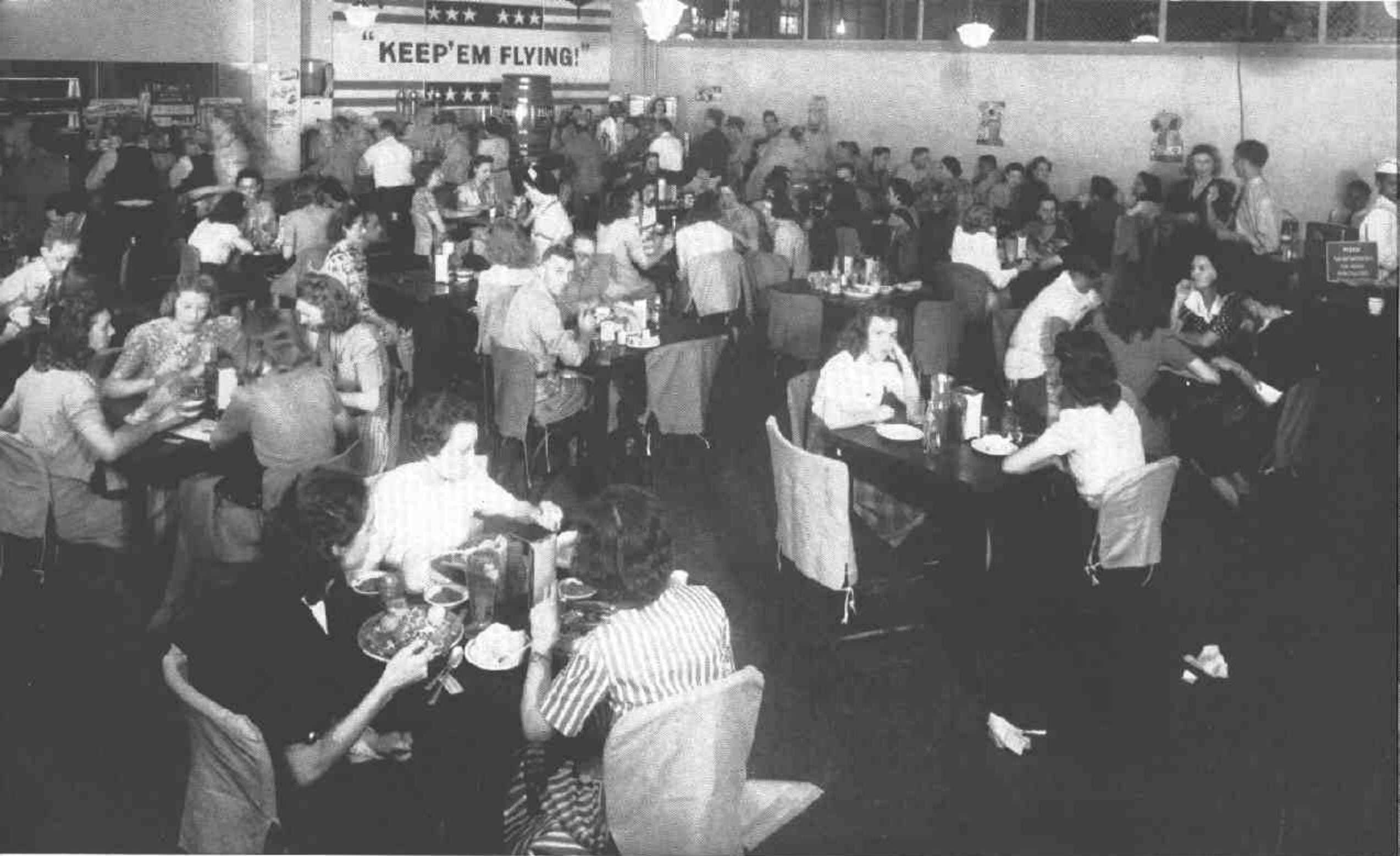
"PX" CAFETERIA, FOR ENLISTED MEN AND CIVILIAN EMPLOYEES
