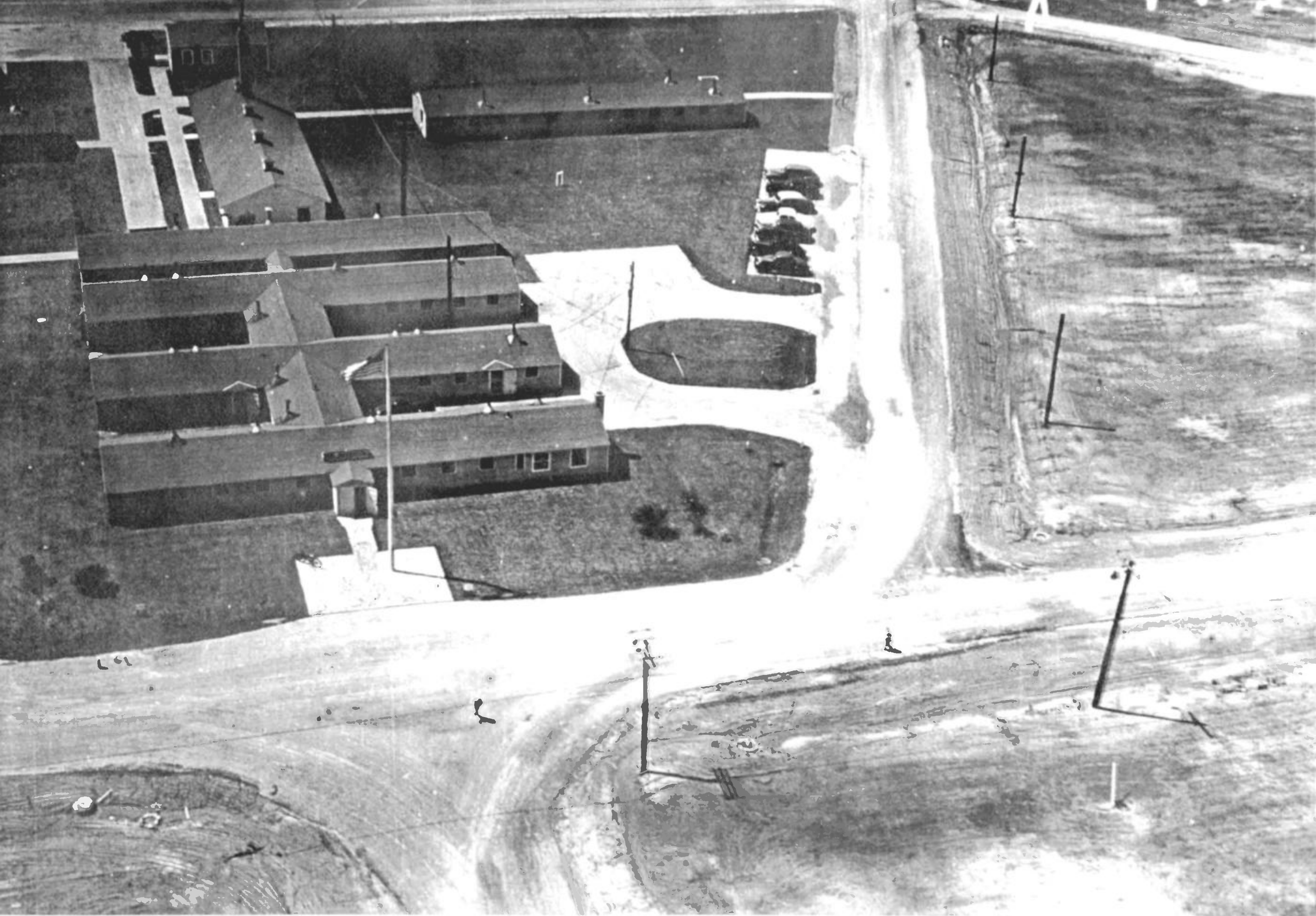
AERIAL VIEW OF FREEMAN FIELD BASE HEADQUARTERS EARLY 1943.
