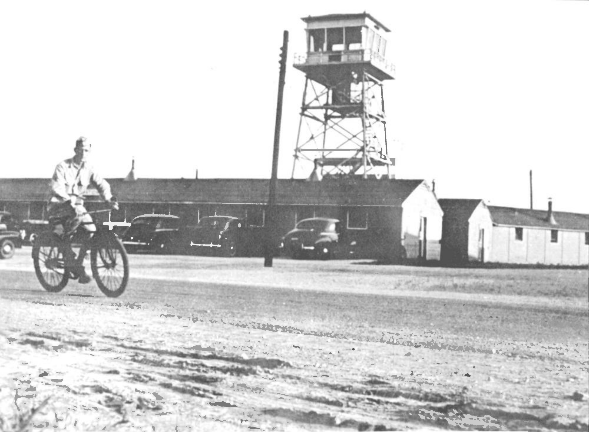
CADET OPERATIONS BUILDING WITH CONTROL TOWER IN BACKGROUND.
