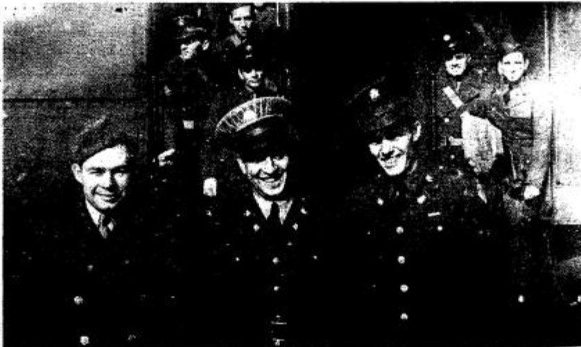
"Hello Seymour". Stepping out of a swollen train on December 8, these first pioneers stood grinning for the cameraman, while others waited anxiously to embark on the task of building Freeman Field; making it another powerful link in the nation-wide chain of flight training stations.
