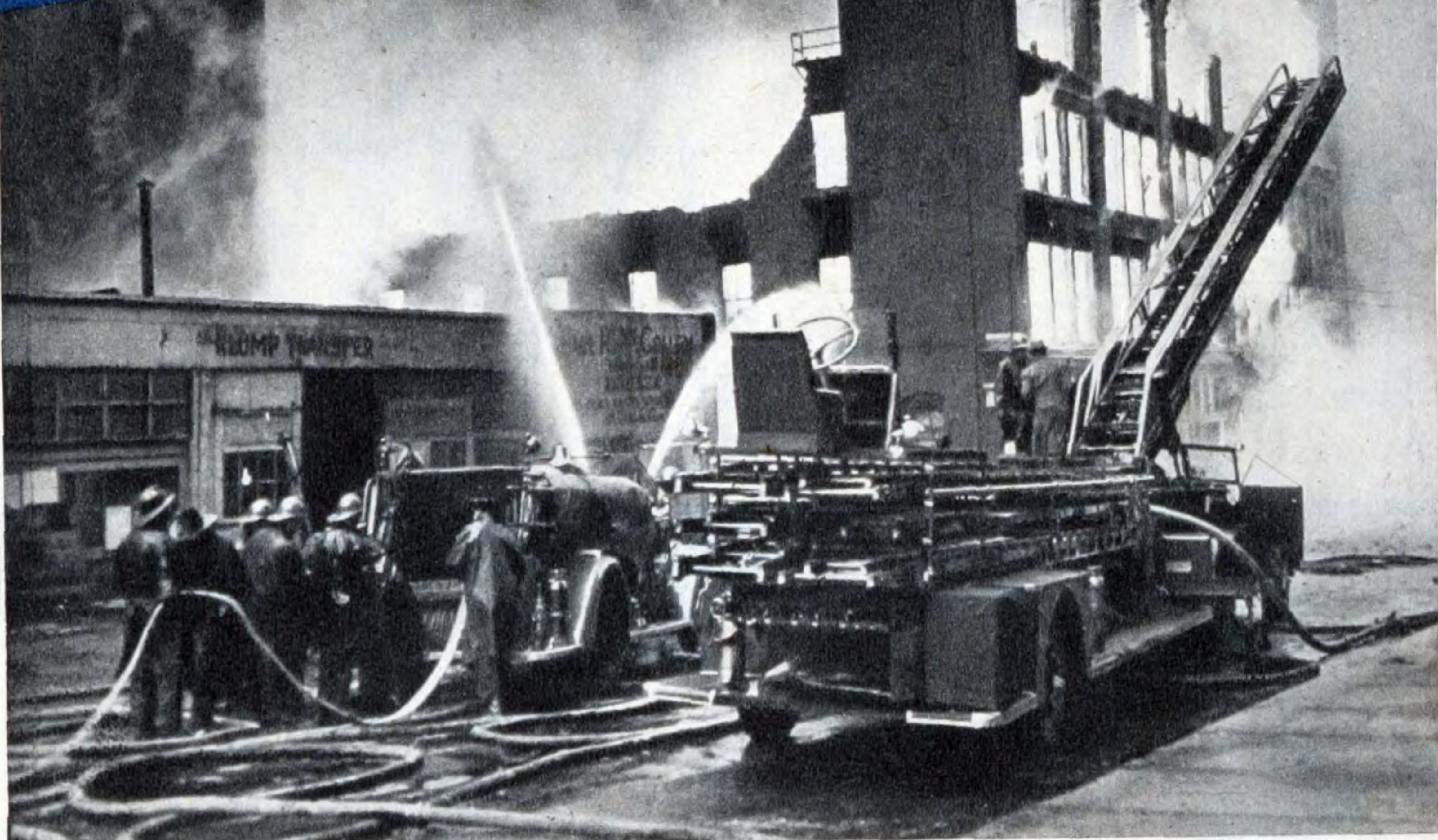
Fires smouldering in a warehouse basement for five hours flared and swept through three buildings in the Kansas City wholesale district. Walls of the building above fell just before the picture was taken.
