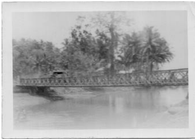
BRIDGE OVER WATER - THIS IS KNOWN AS A BAILEY BRIDGE - OUR ENGINEERS COULD RAPIDLY ERECT THESE BRIDGES
