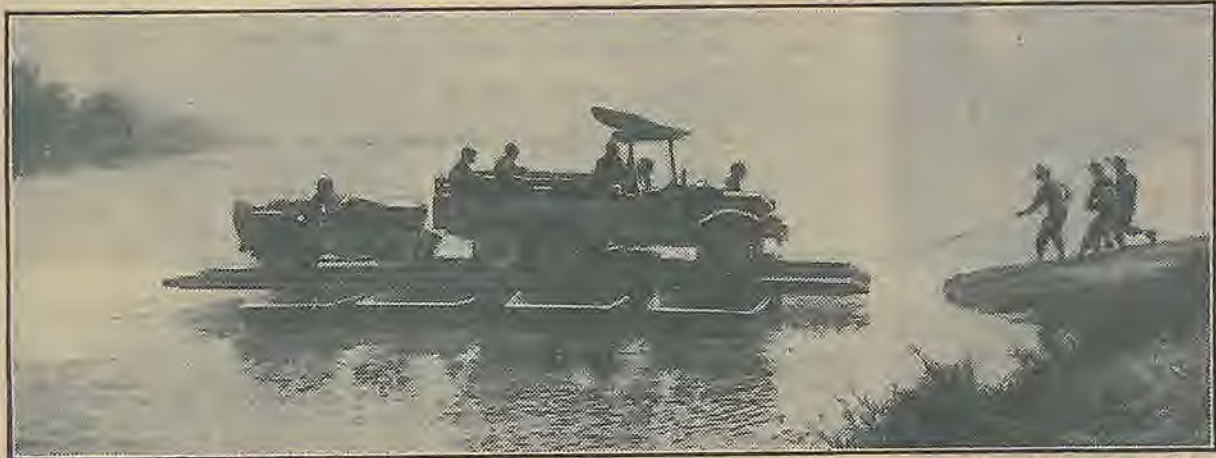
SMOKE SCREEN, against which vehicles being ferried across river are silhouetted, effectively hinders German shelling of crossing site. Here men ashore haul raft in close for fast unloading at good landing place.
