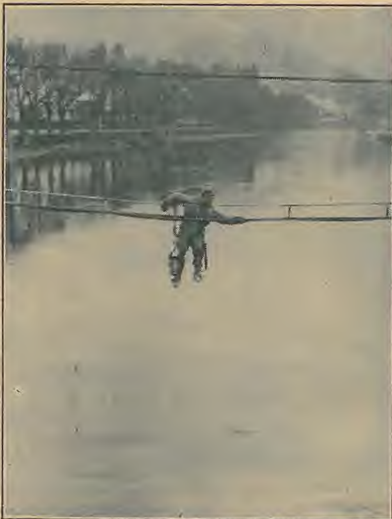
Here's a wireman's own bridgehead over the Moselle. Pvt. Arley Norman, of Newcomerstown, Ohio, crosses by cable-car to check telephone lines over river.
