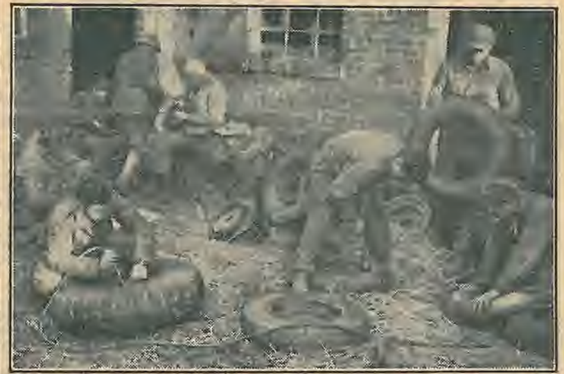
Without tires, supplies can't be rushed to the front—and without supplies, doughboys can't advance on the road to Berlin. Here, somewhere in Germany, members of a tire-repair outfit are shown vulcanizing tires hit by shrapnel. U.K. soldiers can do their part in combating the tire crisis, made known by Gen. Eisenhower, by conducting a personal tire-conservation program.
