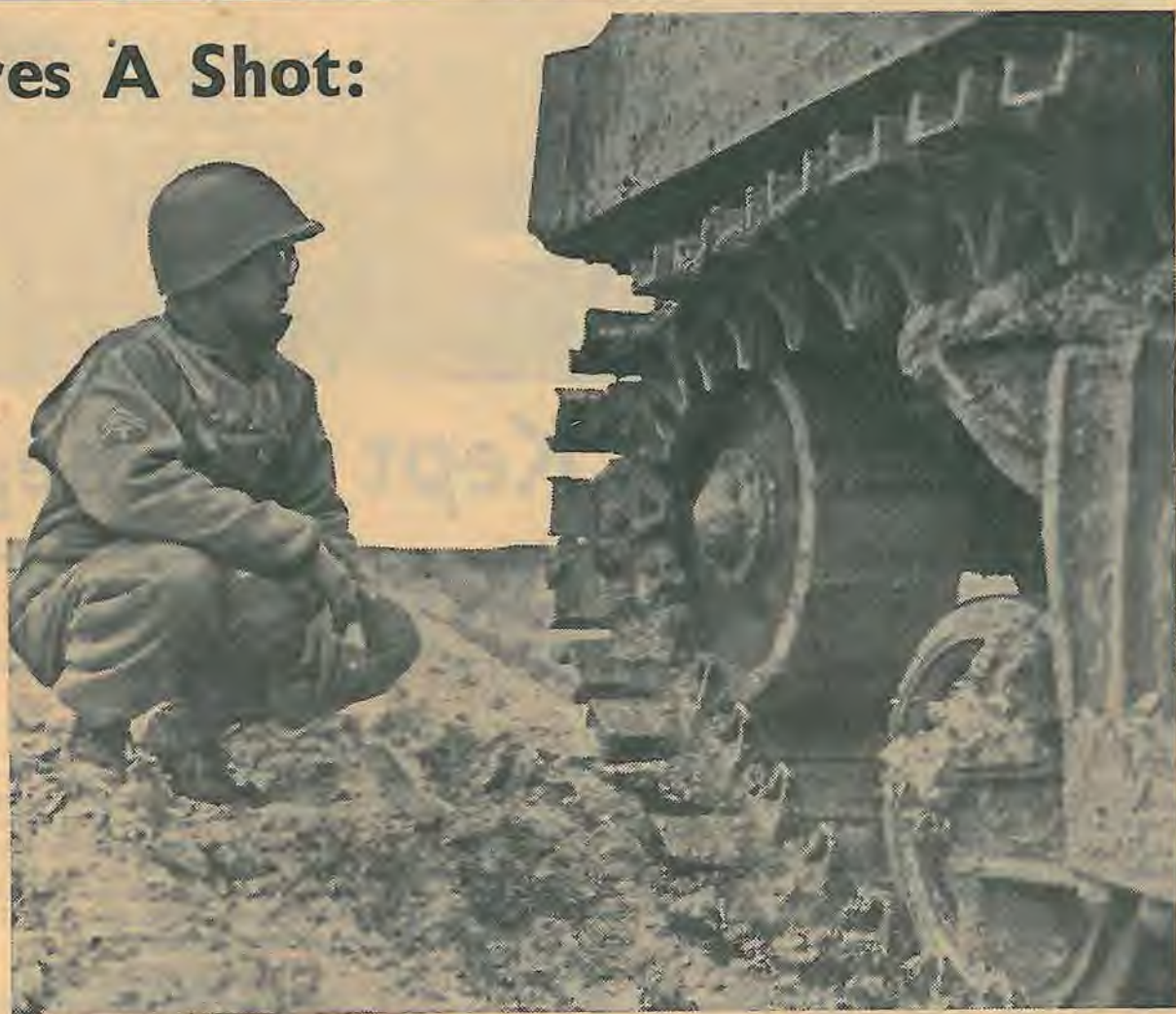
"Duck Bills" on tracks help tankmen pull out of the goo when going gets rough.
