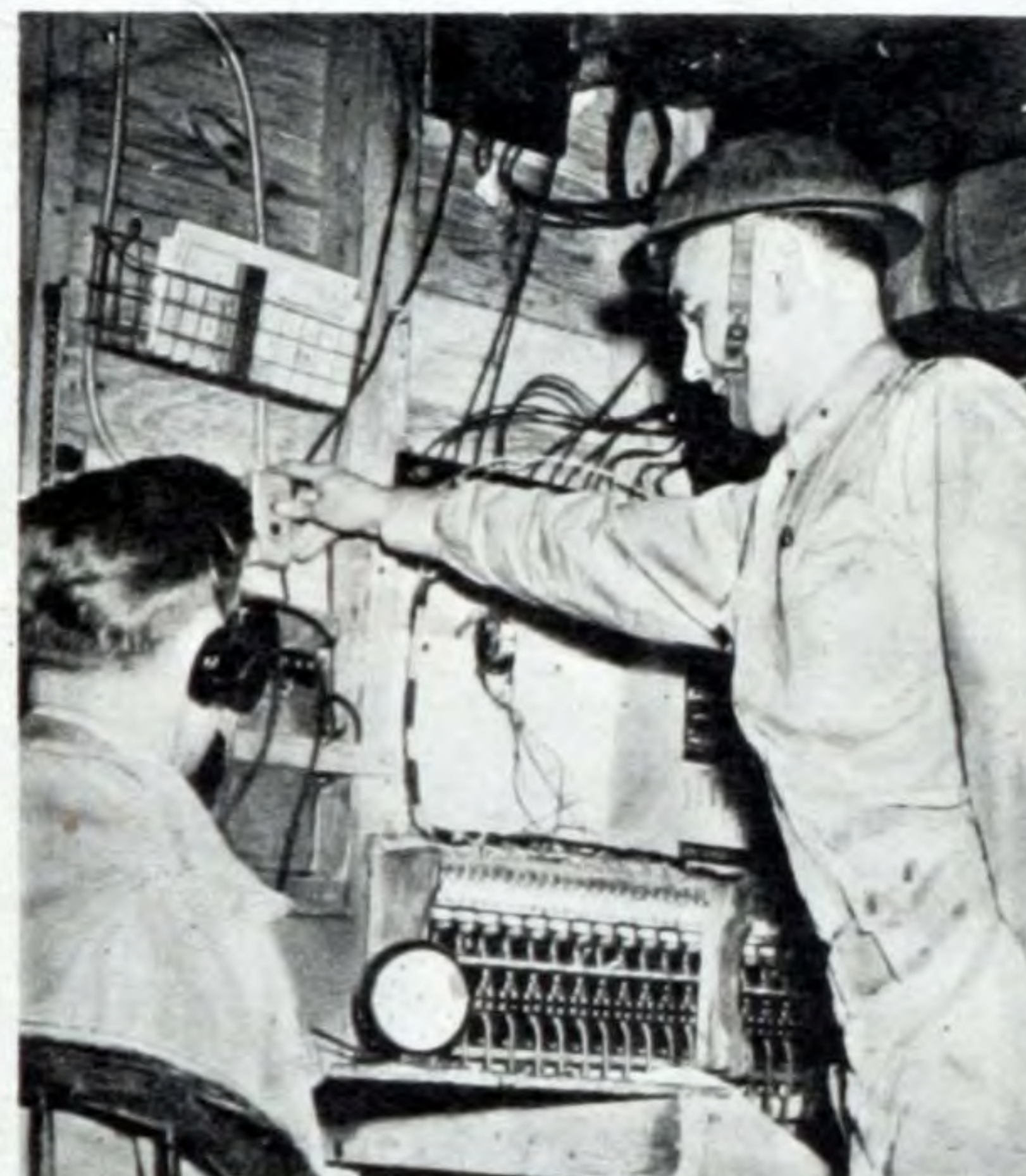
"Hot loop" phone circuit is kept constantly open for alert from spotters.
