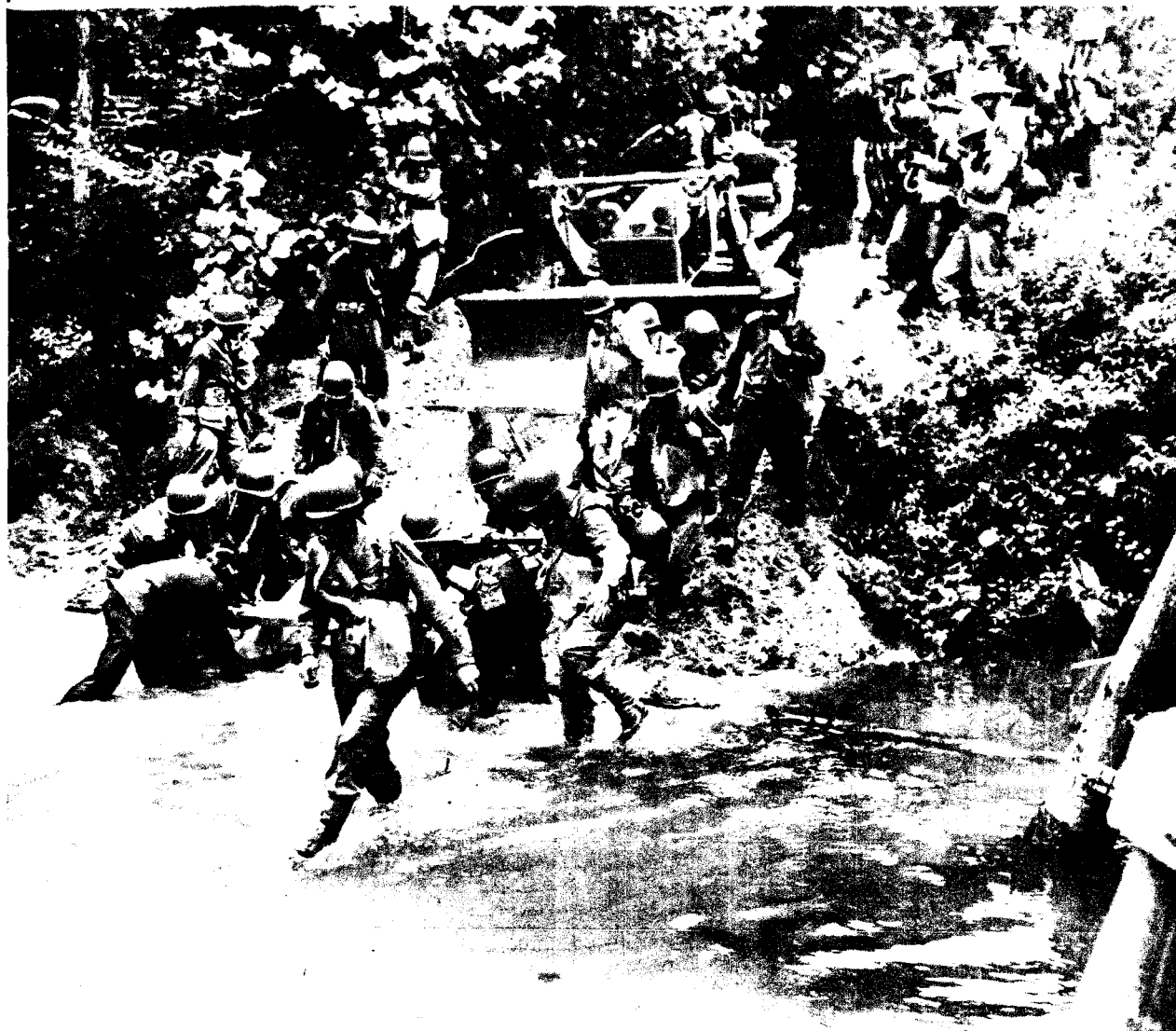
On maneuvers in Louisiana these engineers put a culvert into place in a river, with the aid of a bulldozer. A simulated gas attack accounts for the masks, making the job a little tougher. A few minutes after this picture was taken they moved on to the next obstacle which, you can wager was no less difficult.
