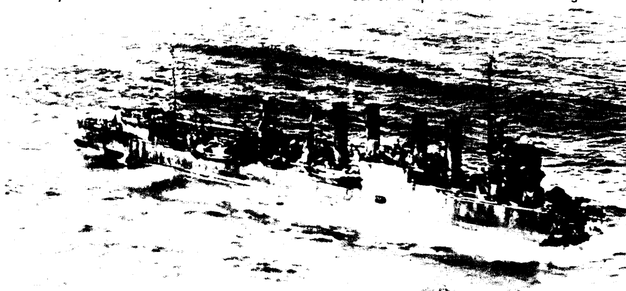
The U.S.S. Blakeley, her bow blown off by an Axis torpedo, managed to plow into a Caribbean port for repairs, then made a 2,000-mile journey to Philadelphia, where a new bow was grafted on her. She's back on the high seas now, in a good shape.
