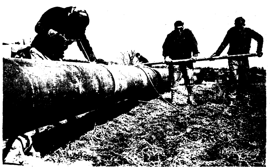
Near Lambertville, N. J., workers weld pipe lengths, beginning the first New Jersey section of the oil pipeline between Texas and New York.
