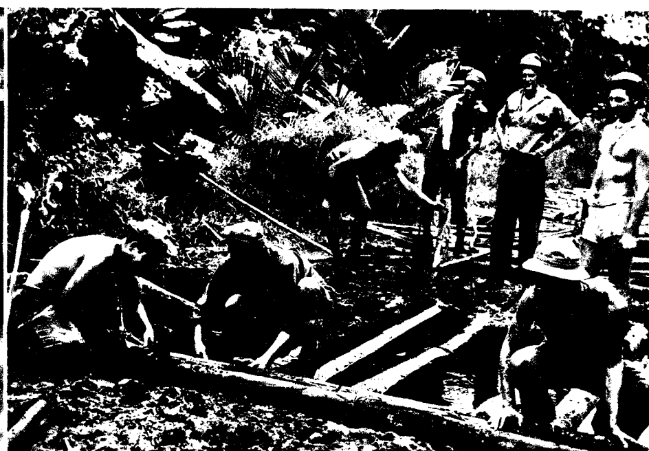
THE ENGINEERS. These GIs are building a corduroy road of cocor palm logs, so that Army supply transport won't bog down in the tropical m
