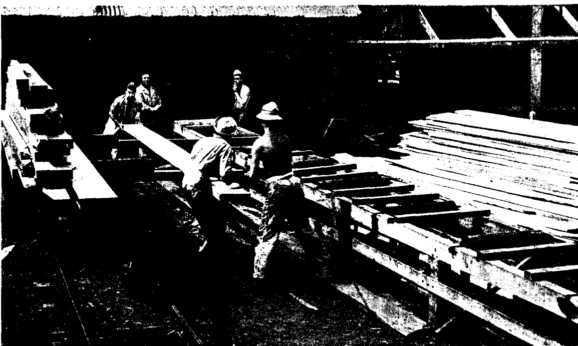
ARMY LOGGERS. Logs come in one end and U. S. soldiers take planks out the other in this Pacific saw mill. Lumber is used for piers, warehouses, barracks.
