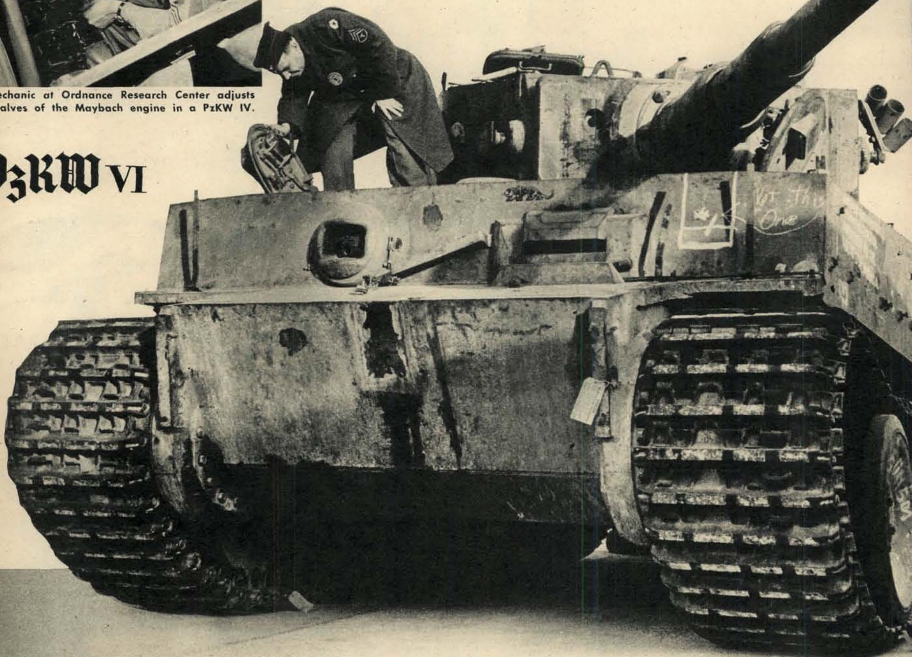
This is the famous Tiger (with a picture of its namesake painted on the face plate), the largest and heaviest German tank. Weighing 61½ tons, it is propelled at a speed of from 15 to 18 miles an hour by a 600-to-650 horsepower Maybach V-12 cylinder engine. Maybach engines are used in many of the Nazi panzer wagen and in submarines. The PzKW VI has an armor
