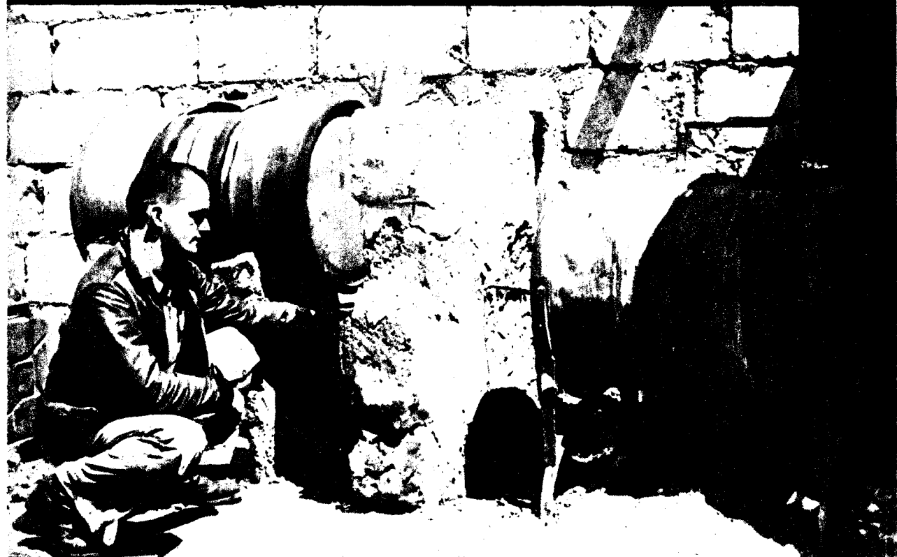
M Sgt. Ray Moyer, who comes from South Fork, Pa., is lighting the hot-water tank so that he and his two pals can enjoy a warm shower. The contraption was built with empty oil barrels and the ever-present Italian stone.
