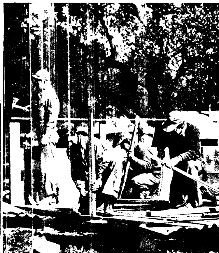
These men are using ballast lumber to construct side walls for the pyramidal tent. Then they'll attach shelves and clothes compartments.
