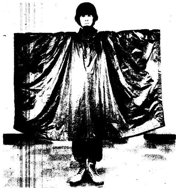
THE ARMY'S NEW NYLON PONCHO for the South Pacific spreads out like this and becomes a shelter half. It can also be used as a foxhole cover, ground sheet, moistureproof bedroll or a raincoat.
