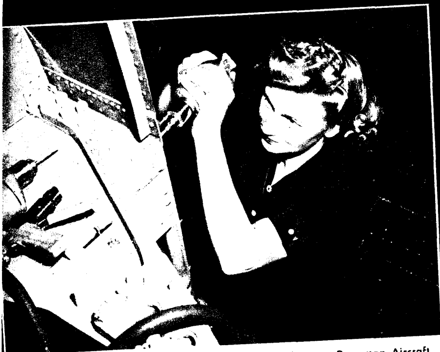
This is a Helicat center section Florence Bruns is drilling at Grumman Aircraft.
