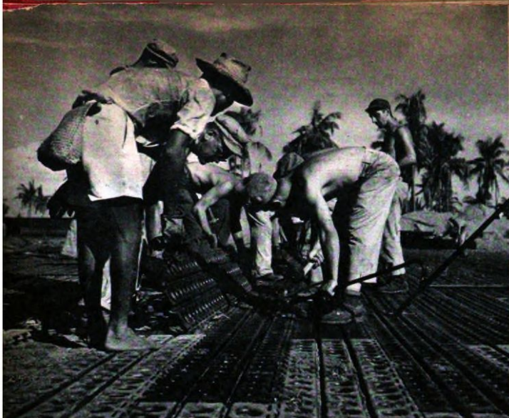
FILIPINOS HELP THE ARMY BUILD ROADS, BRIDGES AND AIRFIELDS. THE NATIVE AT THE LEFT LENDS A HAND TO GI ENGINEERS LAYING A SECTION OF MATTING ON AN AIRSTRIP.
