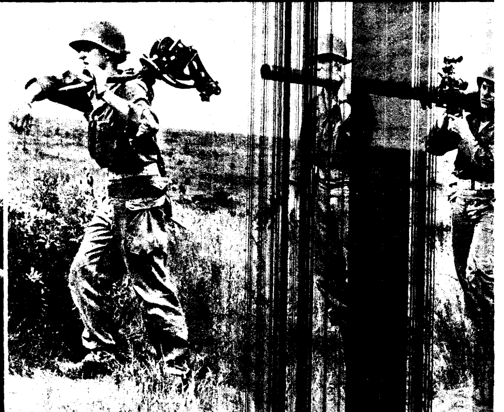
How you can carry the 75-mm. One man has the tripod, two others the barrel.
