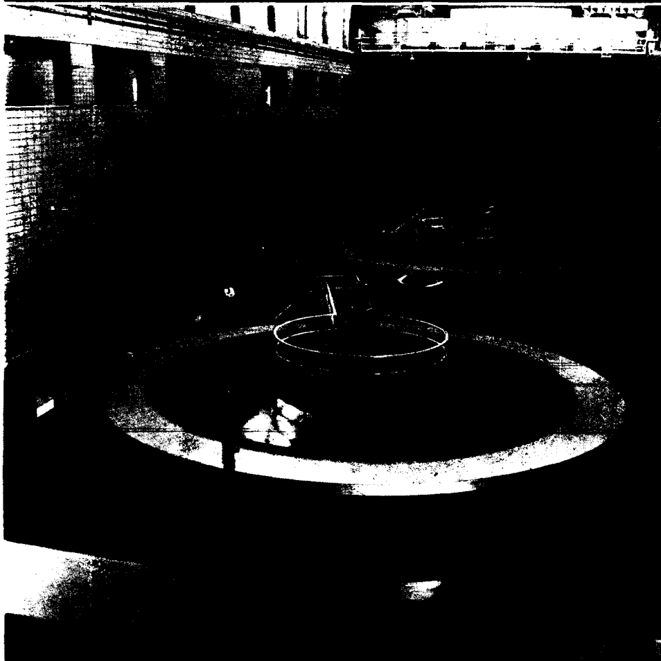
Generators in the power house of Chickamauga Dam near Chattanooga. Each is coupled to a 36,000-hp motor which is turned by water the dam impounds.
